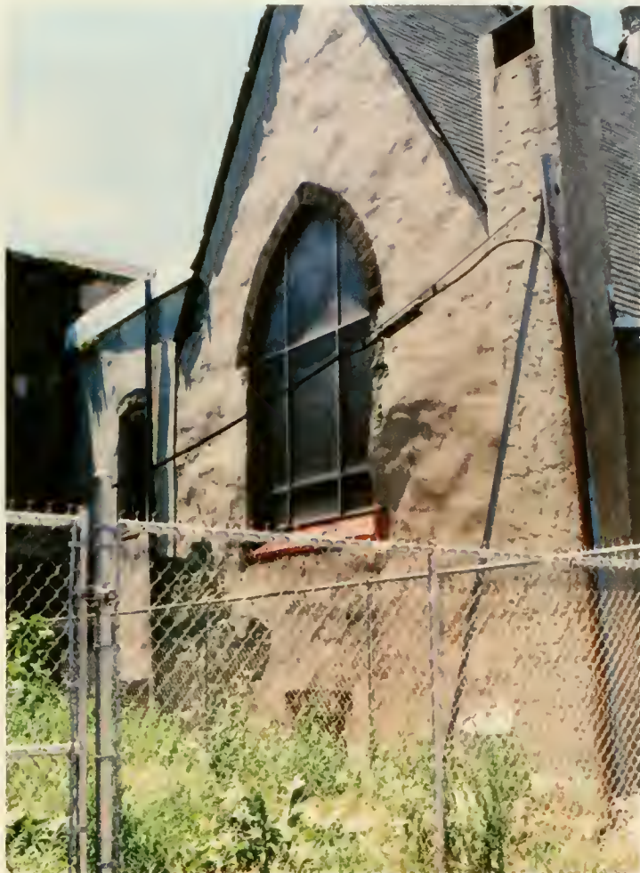
East Elevation of Church Building (Q)
